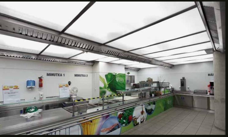
The new CSOB headquarters is the biggest office block in Prague and at the same time biggest building in the Czech Republic and central Europe constructed to ecological standards. TPV ventilation and air-conditioning ceilings are installed in the kitchen and canteens with a total area of 330 m<sup>2</sup>. The canteens use polycarbonate in two layers to ensure the perfect diffusion of light and uniform lighting in the space below the ventilation ceiling.
